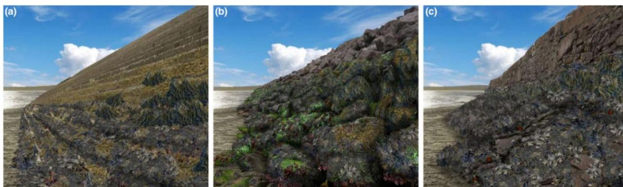
Figure 3 - Examples of images of structures (a-c) used in the survey. Variation in the underlying structures, from stepped walls (a) to rip-rap walls (b) and heritage stone walls (c). Source: Fairchild et al. (2022)
